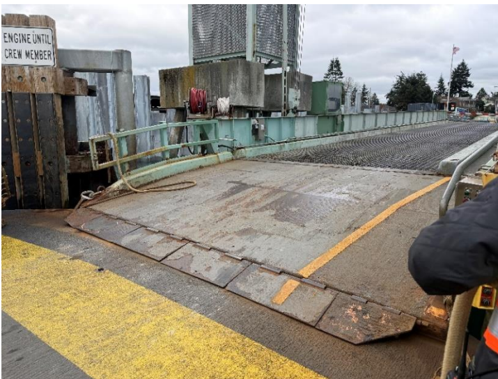
Anacortes Bridge Apron
