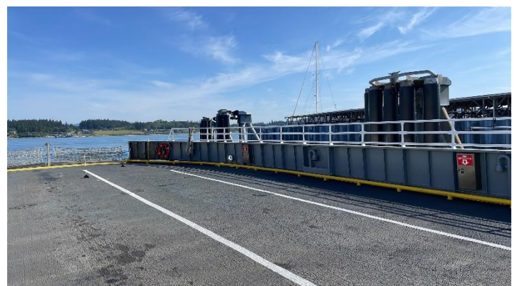
Repainted Ferry Bulwark
